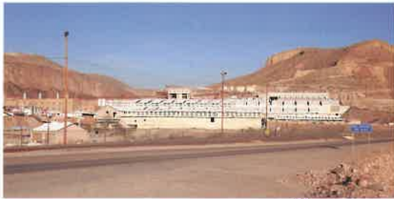
▲ FIGURE 11-14 COPPER MINING AND CONCENTRATION Morenci Mine, Arizona, is the largest copper mine in the United States. Nearby are other bulk-reducing facilities, including the concentrator shown here.
